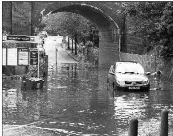
The July 2007 flooding (Photograph by Alan Barnes, Buttermere Gardens)
